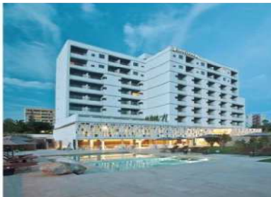
Hotel OD Port Portals Mallorca
