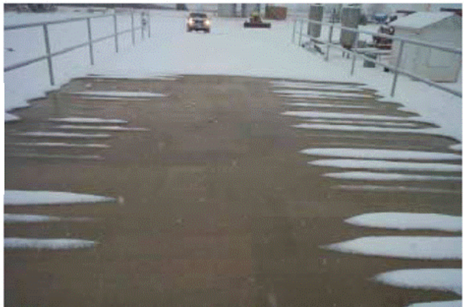
Foto 5.10. Puente Deck en Oklahoma State University, Stillwater, EE. UU. (Fuente: Bose, J.E. et al. Oklahoma State University).
